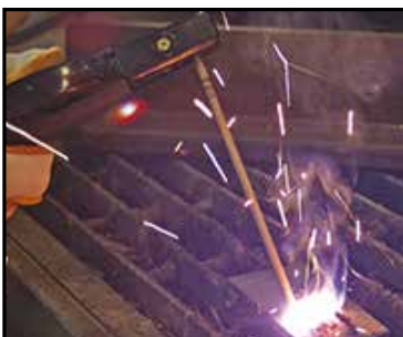
(6) Hold the electrode slightly above the work maintaining the arc while travelling at an even speed.
