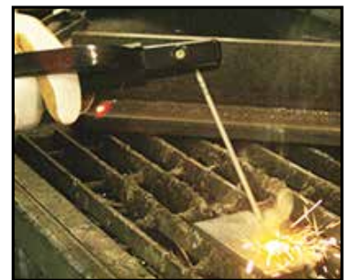
(5) Strike the electrode against the workpiece to create and arc and hold the electrode steady to maintain the arc.
